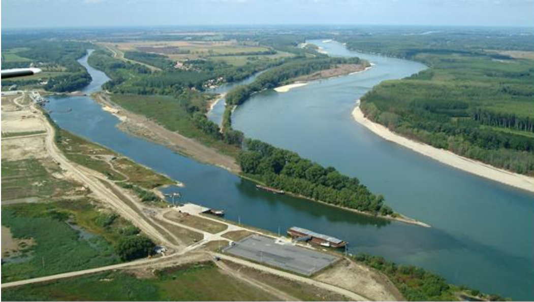
Figure 31: Before the construction works started at Mosoni-Danube and Danube estuary section
