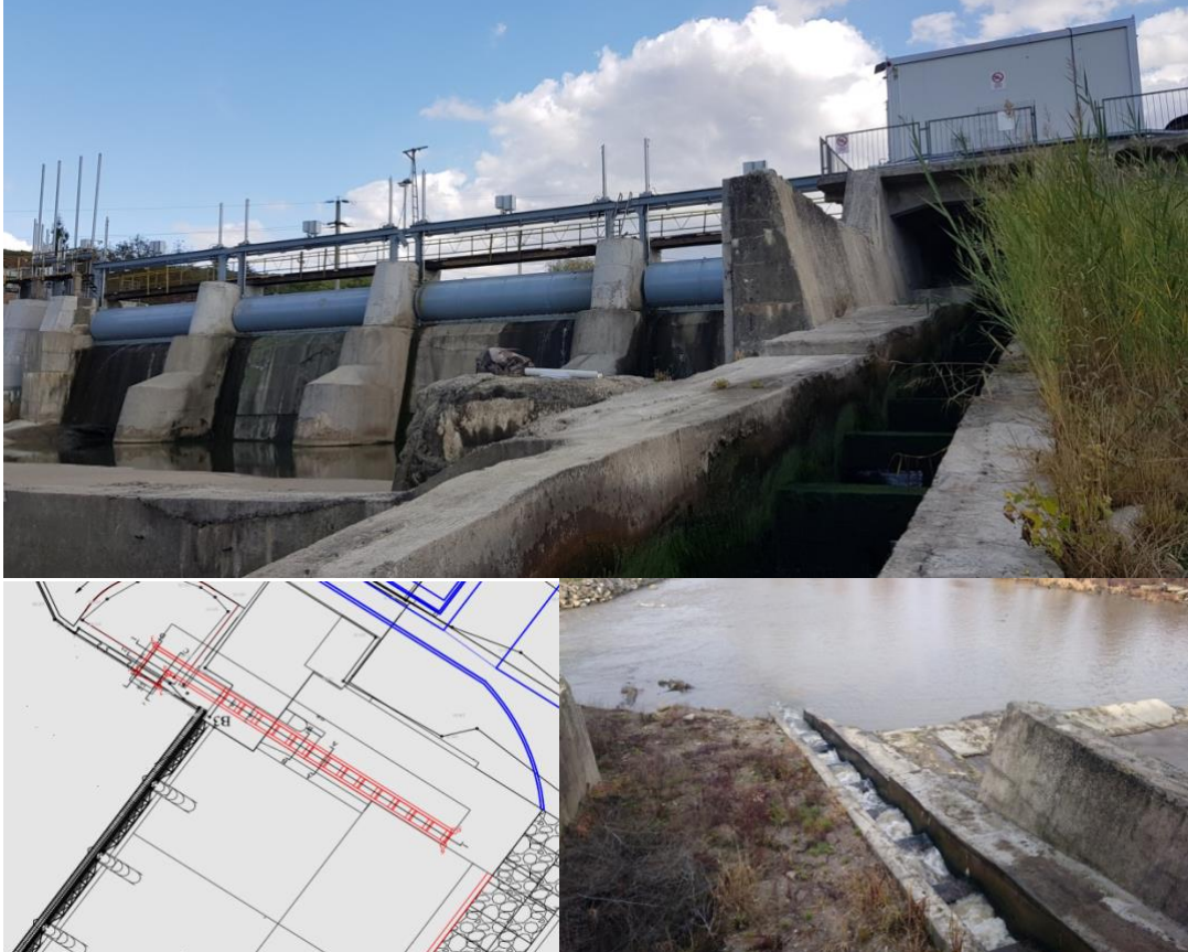
Figure 25: Construction scheme / Photo - fish pass
