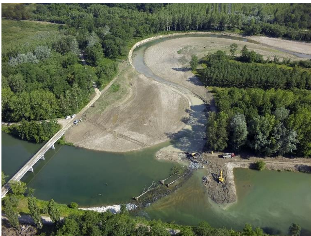
Figure 2: Construction works in the Traisen-area ©Verbund
