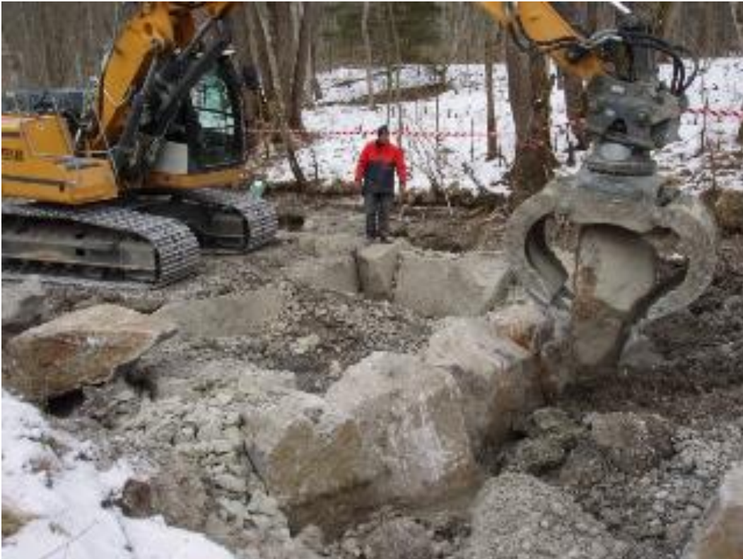
Figure 8: Construction of the measure
