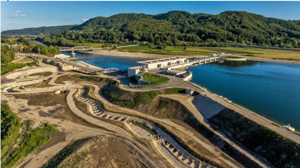
Figure 33: HPP Brežice and the fish pass on the Sava River after construction
