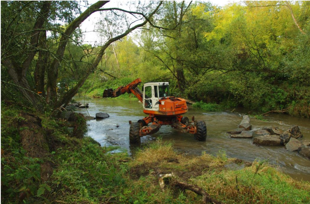
Figure 21: Inappropriate bank lining were removed and used for initiation elements
