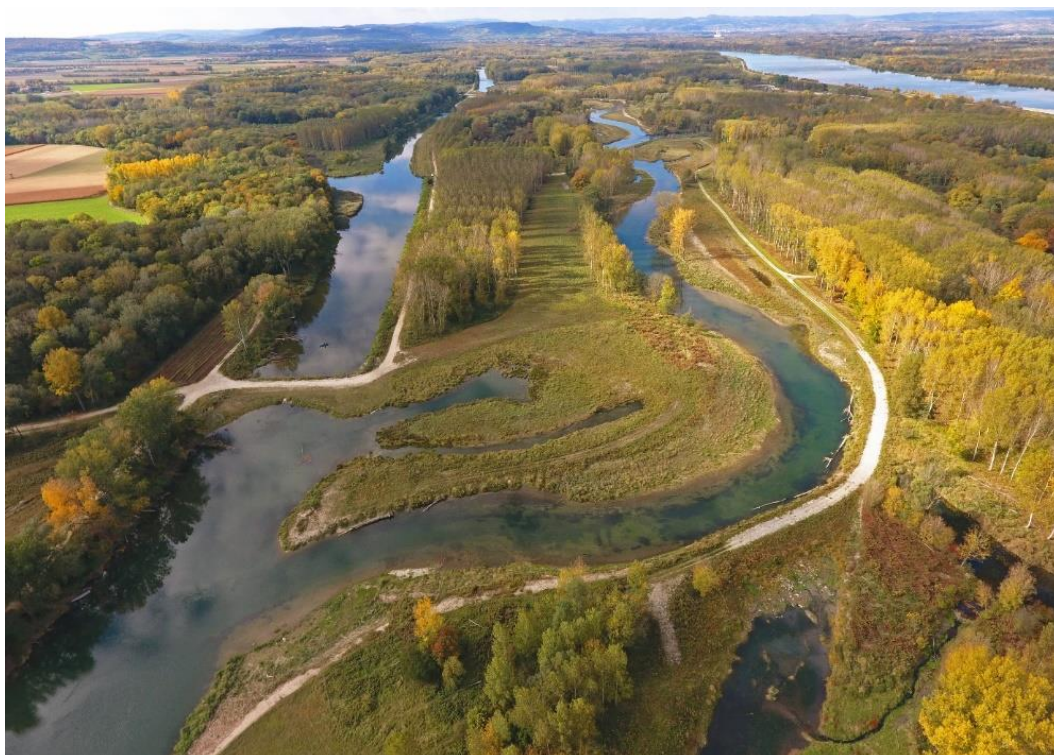
Figure 3: Restored section of the Traisen River, next to the Danube River (upper right) ©Verbund
