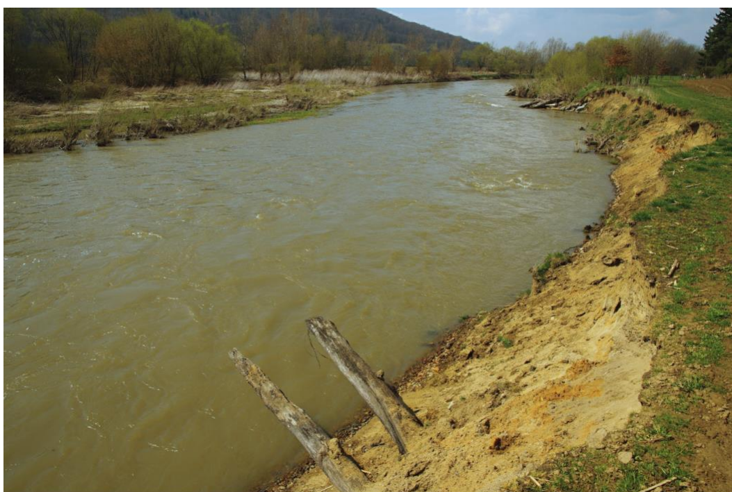
Figure 19: In some places it was necessary to correct the development of nature-friendly river bed interventions
